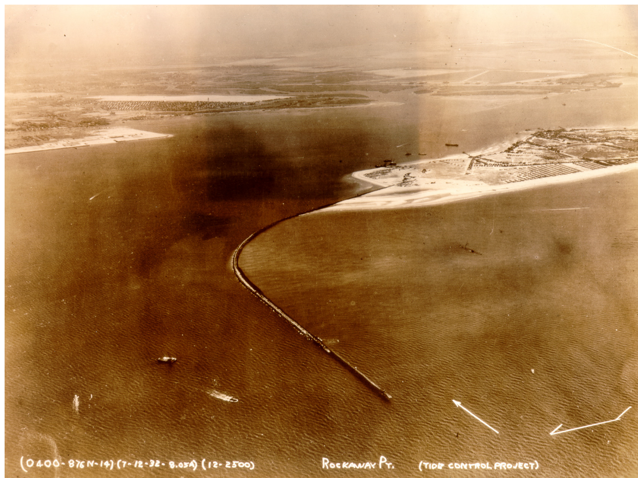
Figure I-3-7. Construction of the jetty on the east side of Rockaway Inlet, Long Island, New York, 12 July 1932. The urban area on the opposite side of the inlet is the east end of Coney Island, and Jamaica Bay is in the distance. In seven decades, the fillet has filled with sand to approximately the end of the jetty seen in this image. Photograph from Beach Erosion Board Archives.
